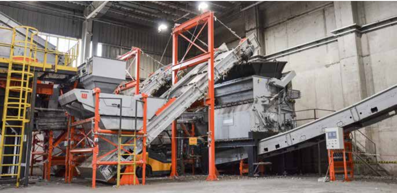
2x PowerLine 3000 with hydraulic drive, Poland
